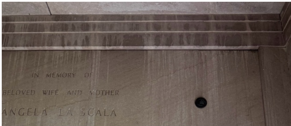
Figure 17: Anisa Estrada, Condensation Detail, 2025.
