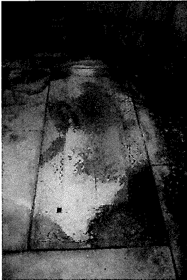
Appendix VIII : Detail of marble crypt covering and stage of deterioration.
