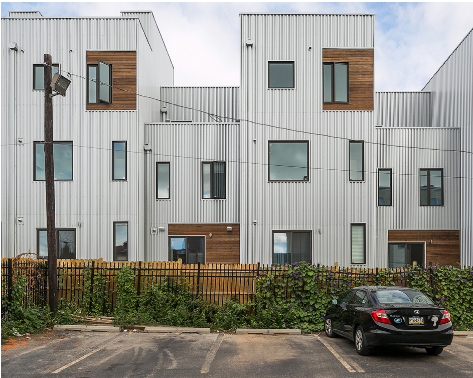
Project selected materials: Brick, metal panel, thermally modified wood Interface Studio Architects
