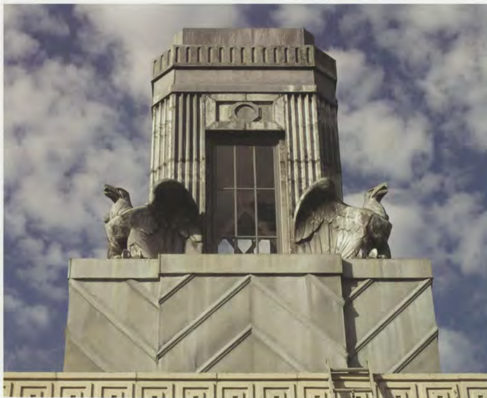
Fig. 4. Ferry Terminal, Ellis Island, lead cupola. Lead experienced a brief revival in the 1920s and 1930s and saw use in some Art Deco and Modern buildings. Photograph by Christopher Barnes, courtesy of Save Ellis Island Foundation.
