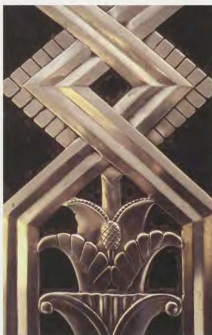
Fig. 2. Chrysler Building, New York City, cast stainless-steel ornament. Stainless steel remains bright without significant treatment but can develop self-sustaining pitting in areas of soiling and must be cleaned periodically. Photographs by the author, unless otherwise noted.
