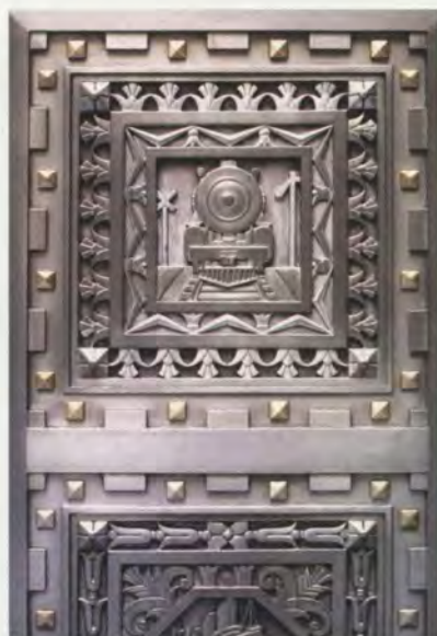
Fig. 5. 20 Exchange Place, New York City, detail of nickel-silver doors, which have not been maintained. Nickel silver in exterior installations will patinate to a dull brown if not maintained with polish and a lacquer finish.
