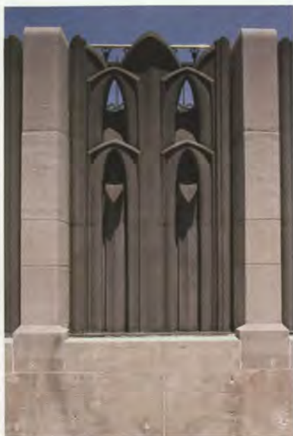
Fig. 3. 30 Rockefeller Center, New York City, cast-aluminum panel at viewing deck. Cast aluminum was used for spandrel panels at the Empire State Building and the towers at Rockefeller Center. Anodic "deplating" was a common treatment for early architectural cast aluminum.
