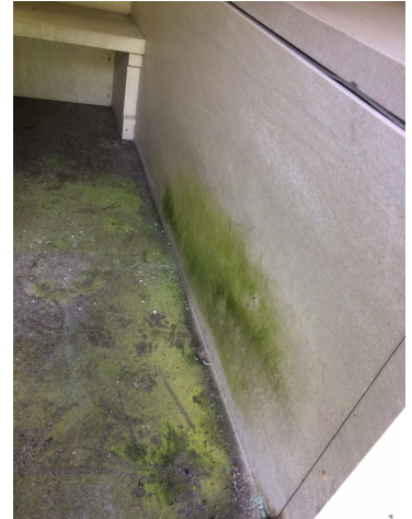
Fig. 13 Biological growth on floor & side of Mrs. Eidlitz's sarcophagus
