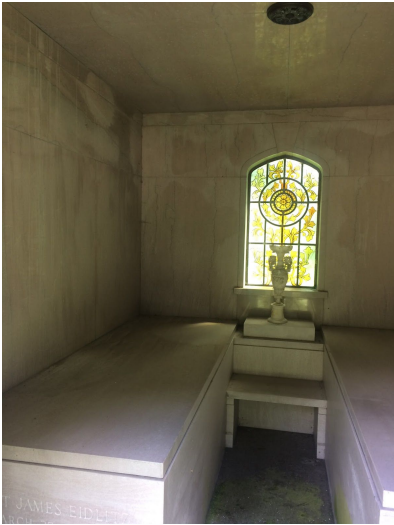
Fig. 8 Interior of Eidlitz Mausoleum, Tennessee Pink "Marble" walls
