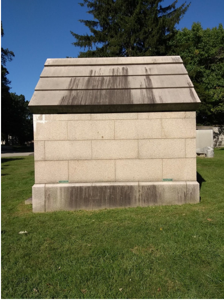
Fig. 10 Side elevation of mausoleum, with conditions visible (biological, lime mortar deposits)
