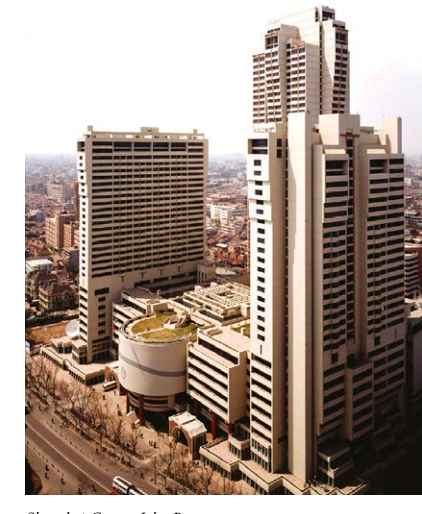
Shanghai Centre, John Portman Shanghai, 1990
