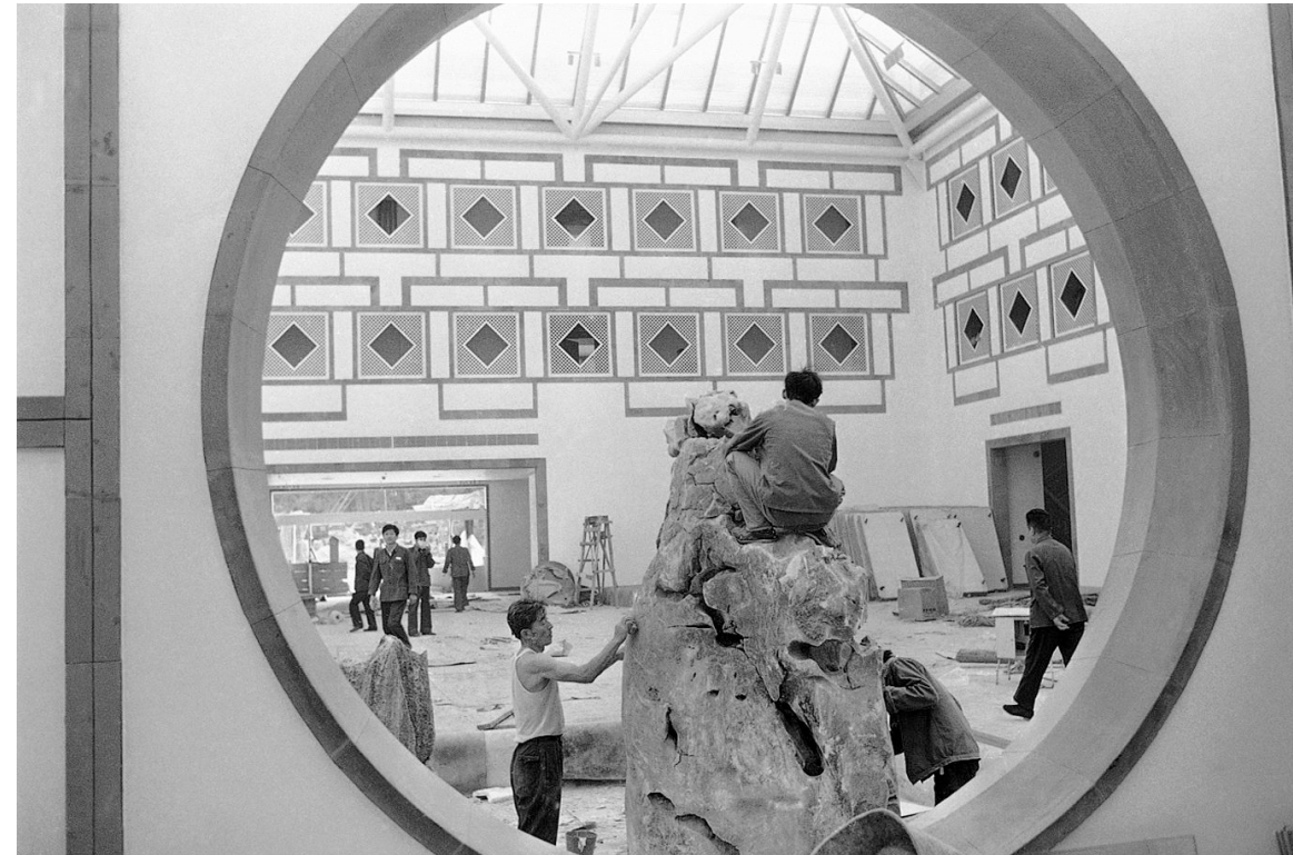
Xiangshan Hotel atrium under construction
