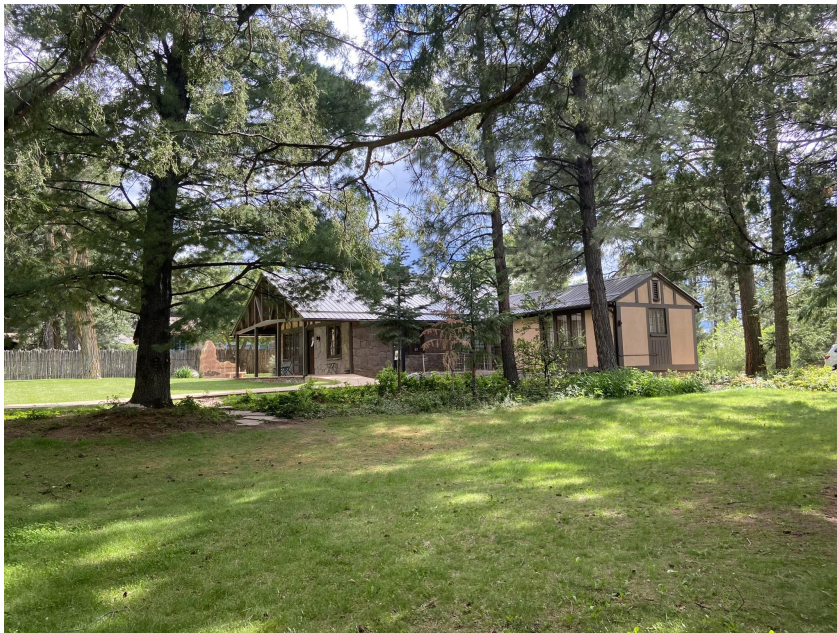
The Oppenheimer House, July 2022. The top photo was taken with an iphone, the lower photo was taken on film.
