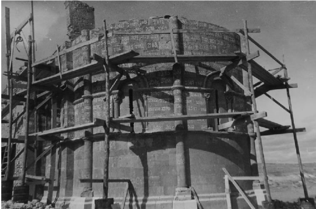
Fig.5 Apse Dismantling. The MET Archive
