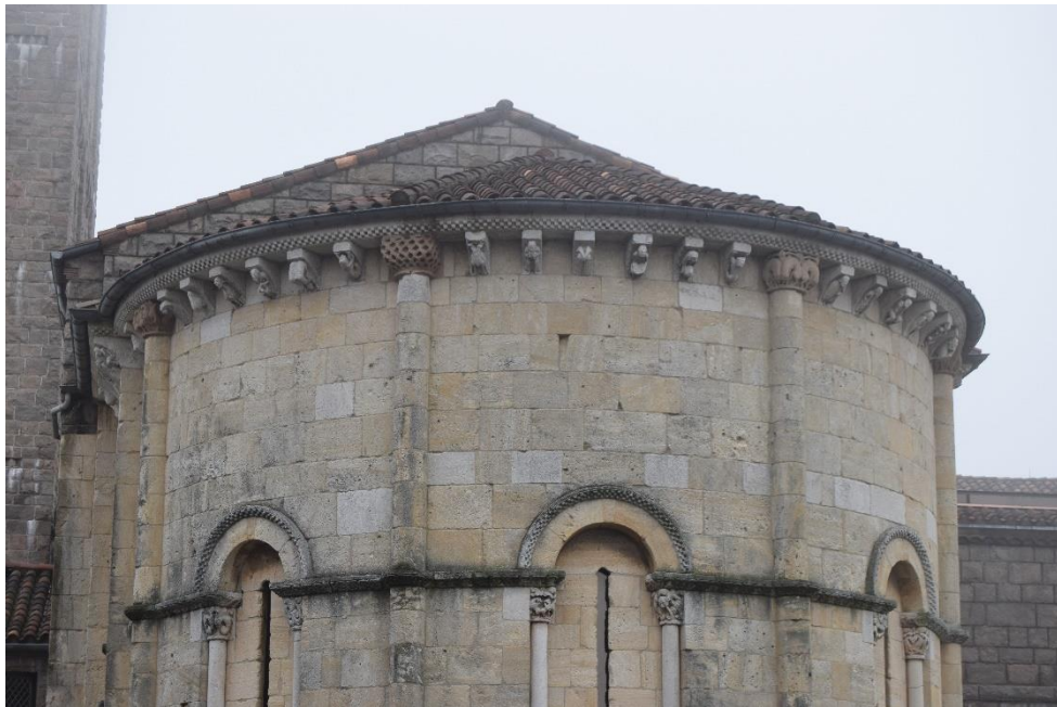
Fig.12 The Apse of San Martín at the MET Cloisters, details (columns and capitals, corbels, windows). Own Resource
