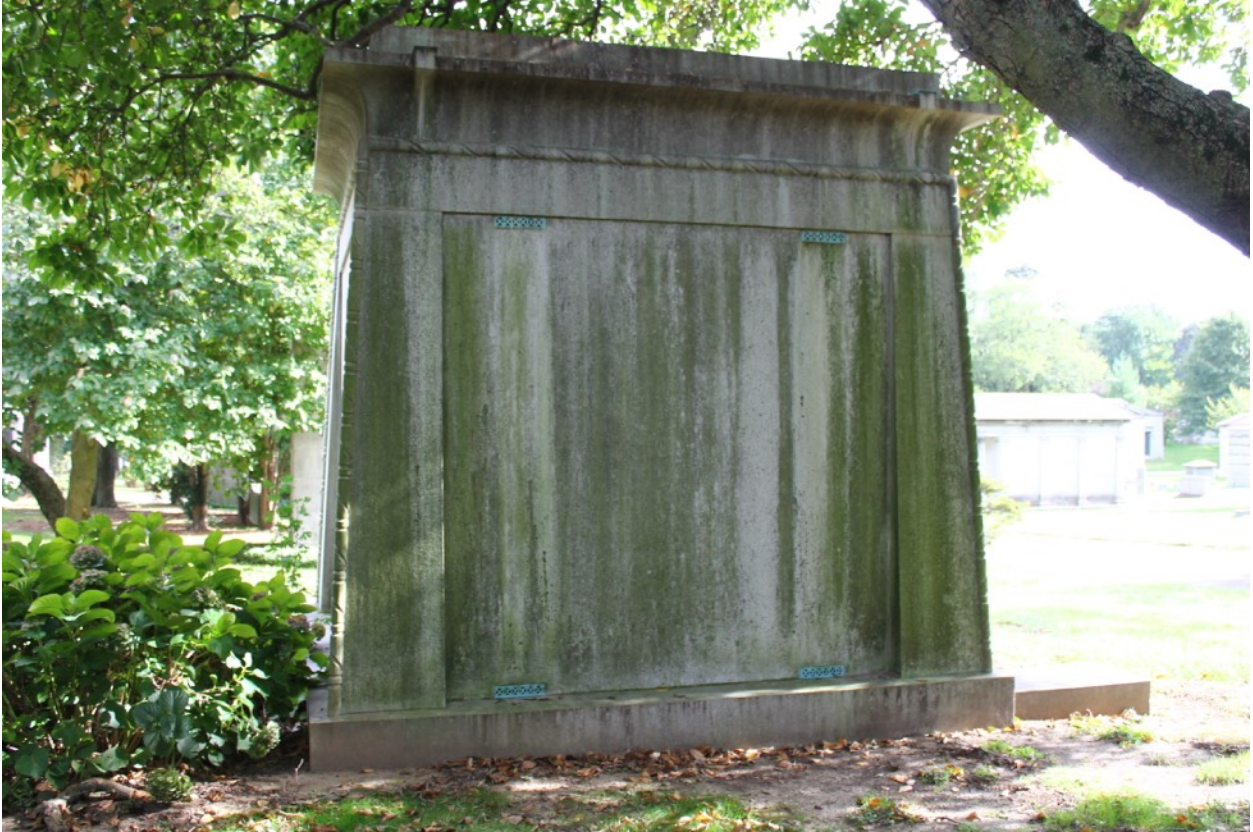
Figure 8: Absence of biological growth beneath copper-containing ventilation grilles.
