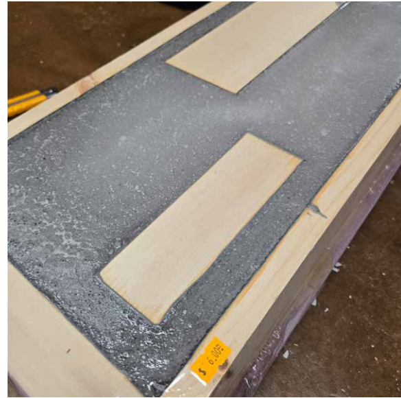
CONCRETE POURING FOR “FOOTING”
