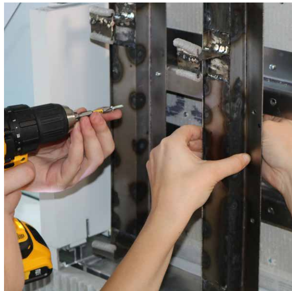
INSTALLING “BRACKETS” TO HANG FACADE
