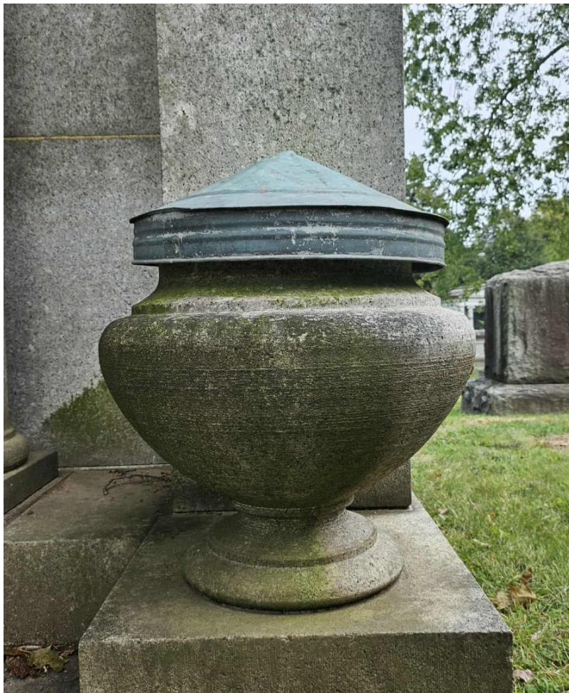
Image 18. Stone urn with copper lid. The urn which is also carved Stonington Pink granite exhibit dampness and biological growth.
