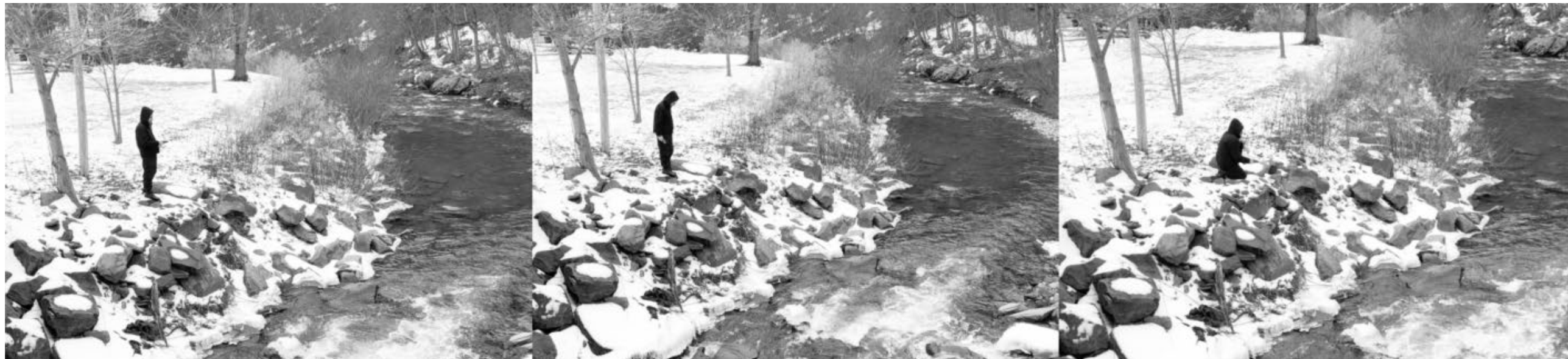
Locals, hikers, pilgrims each carry one stone from quarry waste along the trail to put into empty gabion wall. Slow but incremental process
