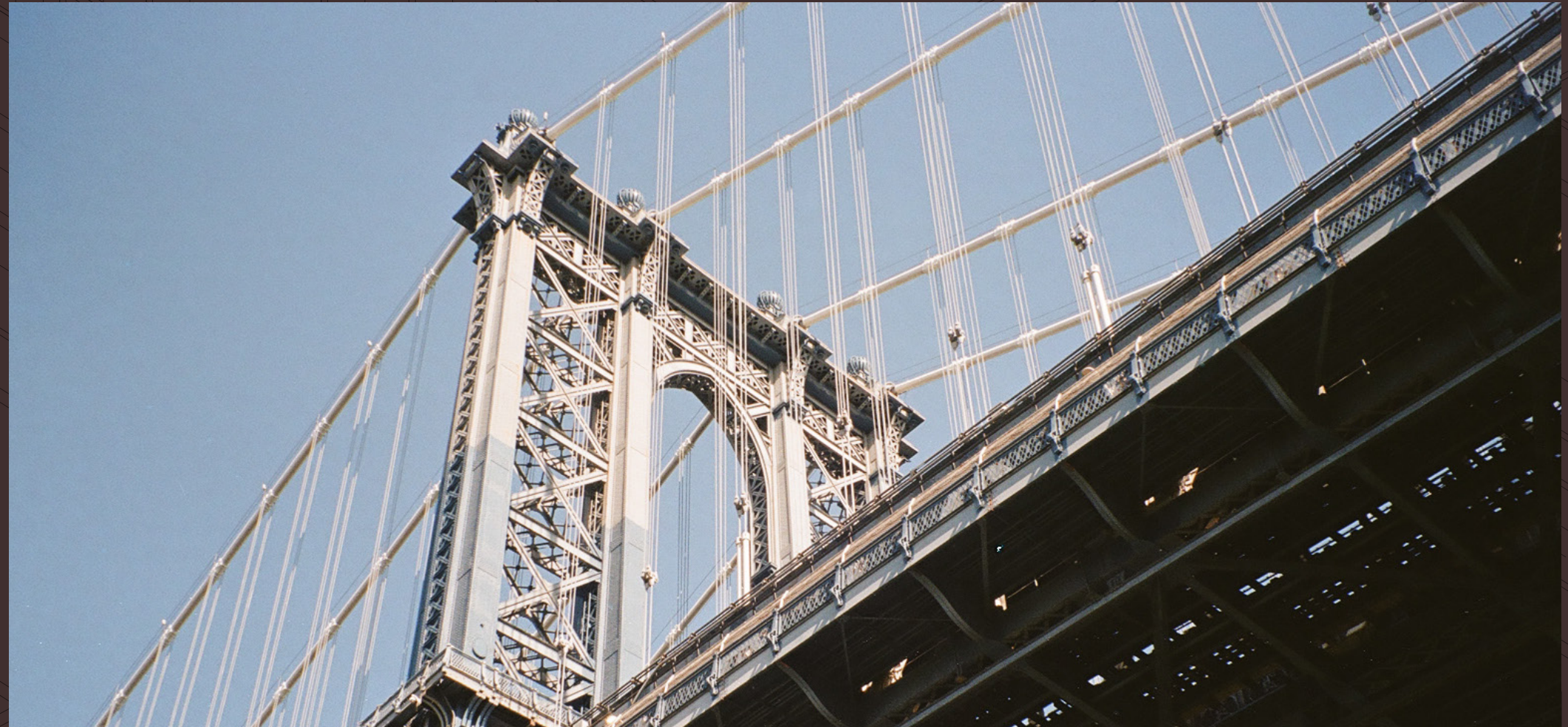
Manhattan Bridge, 20 October 2023
