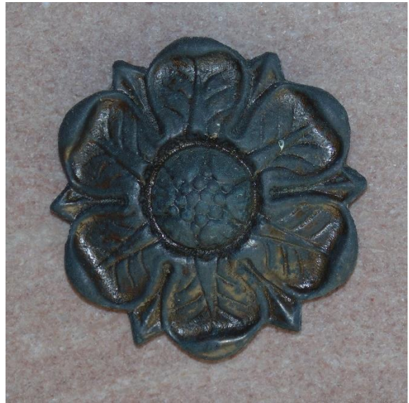
Figure 12: Detail → Cast Bronze Rosettes
