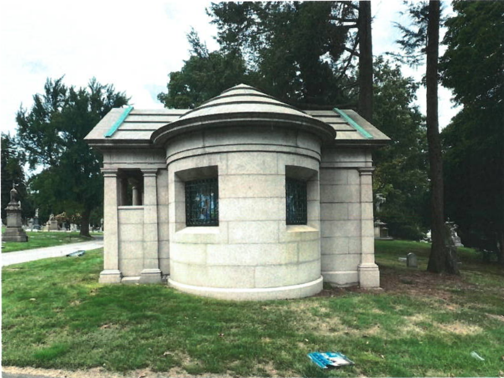
Figure 5: Santana-Miranda, South façade of Fayerweather Mausoleum , 2022.
