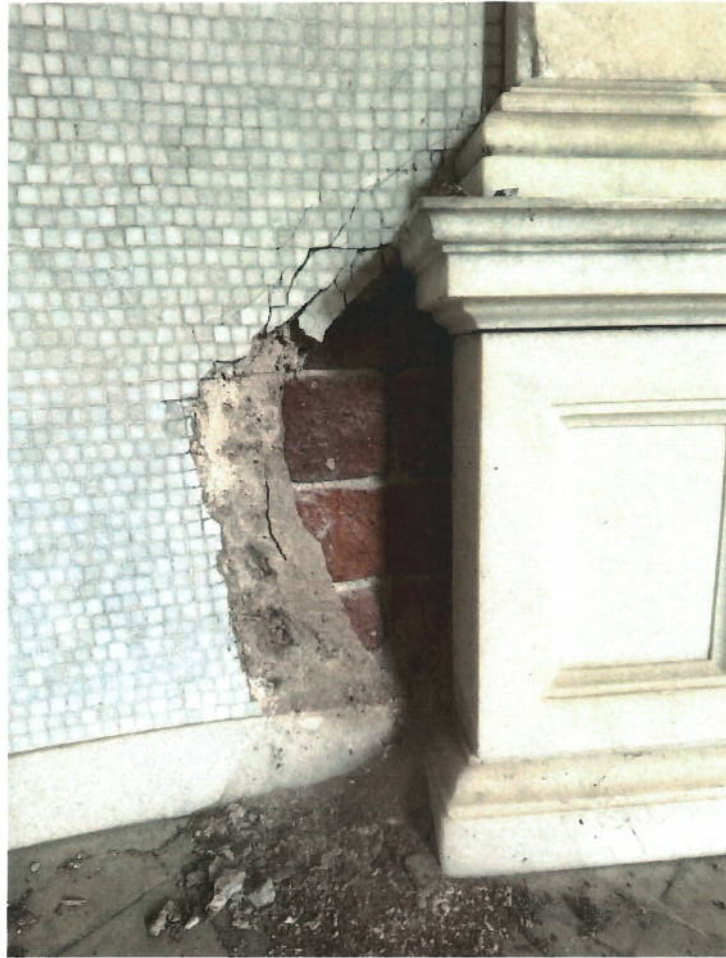
Figure 12: Santana-Miranda, Decay of mosaics demonstrating brick masonry course , 2022.
