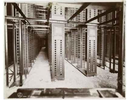
Load bearing stacks under the NYPL
