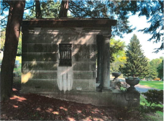
Figure 2: Phetteplace, West Elevation , 2022.
