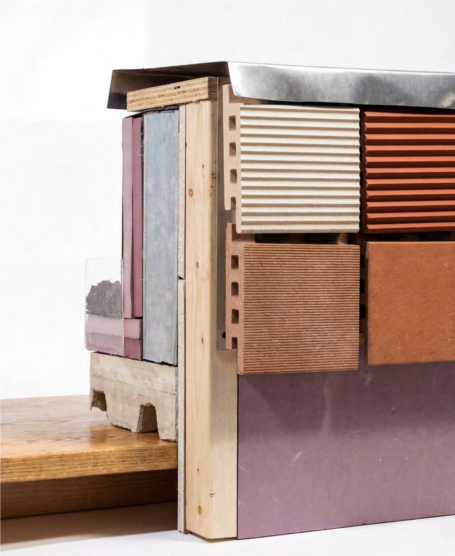
1:1 Physical Mock Up | Terracotta Cladding Facade | Group Work
