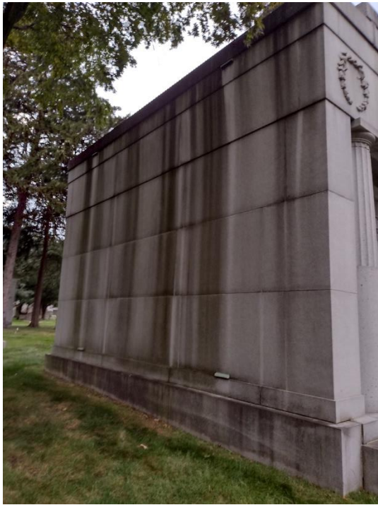
Figure 6: outh Elevation showing biological growth
