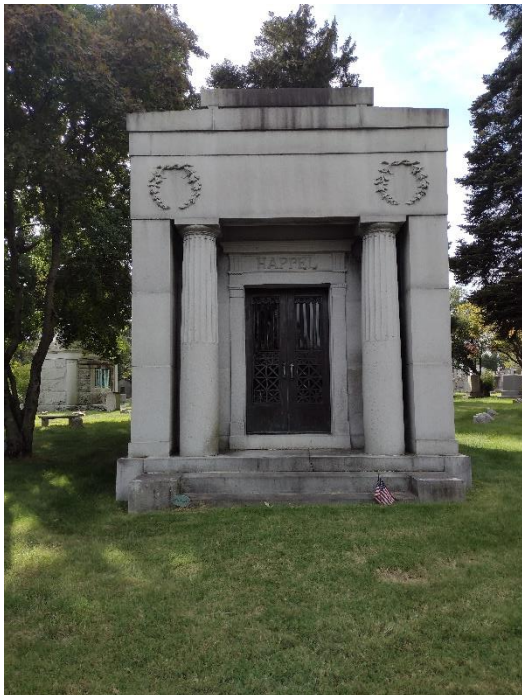
Figure 1: East Elevation of the Mausoleum
