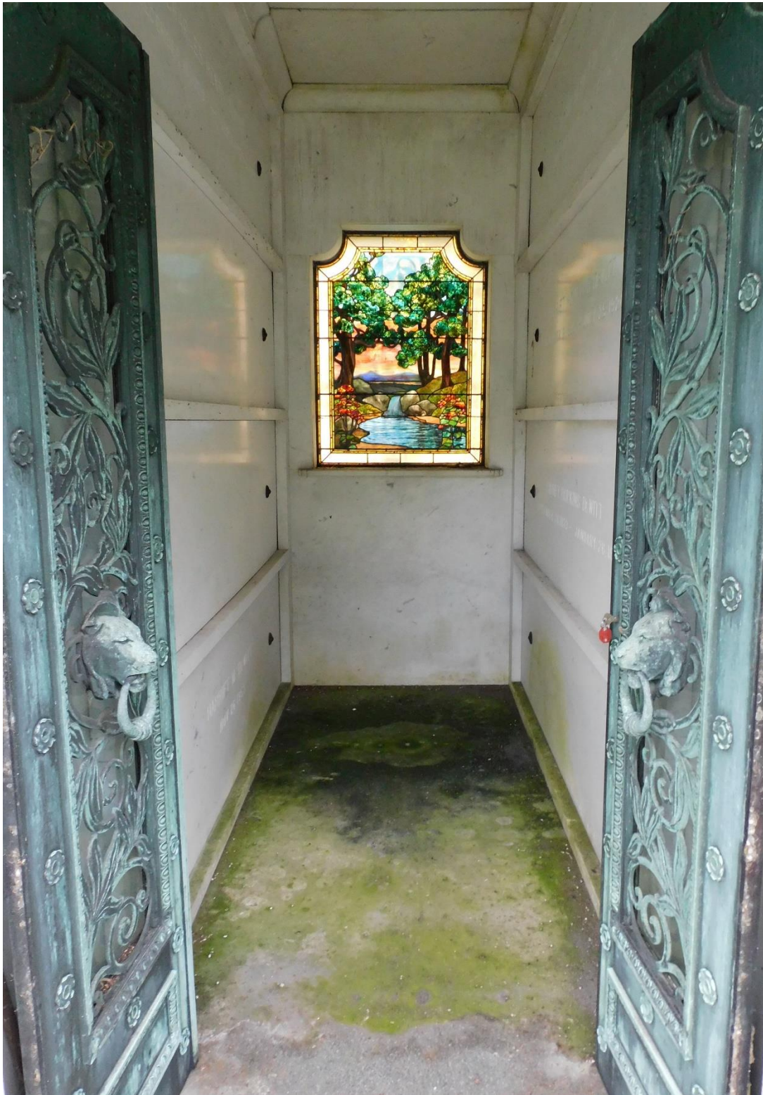
Figure 7: Conditions Detail 1, interior biological growth
