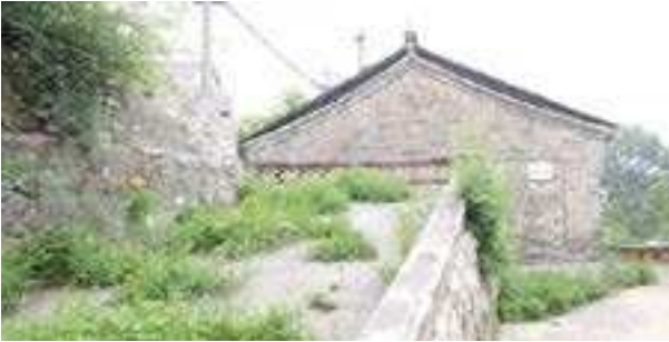
Photo of the West Elevation
