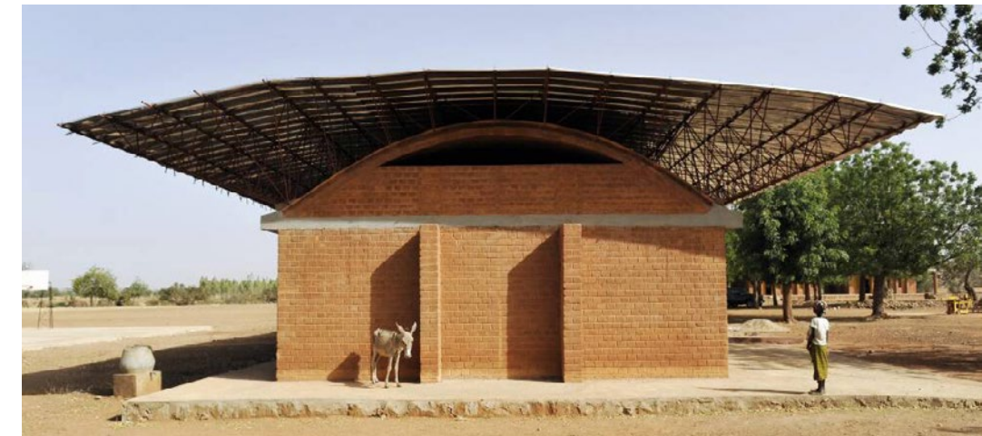
Gando Primary school extension (Photo sourced from Dezeen)
