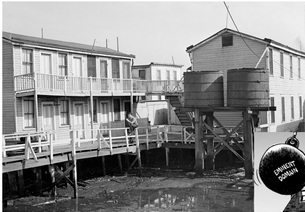
Houses built on stilts over swamp land, Barren Island, Brooklyn, 1937. Photographer: Edwards. WPA Federal Writers' Project Collection, NYC Municipal Archives.
