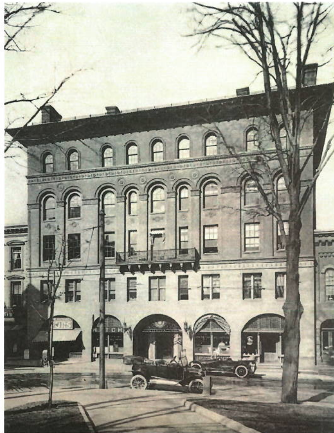
Figure 1: A view of the building at East 76th Street in New York City, designed by McKim, Mead & White, 1870-1871. (The drawing was reproduced in "The City of New York" by George C. Fox, 1924. Copyright © 2014 Avery Library.)
