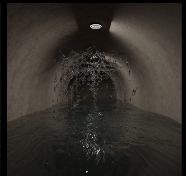
N50 - Water Chamber
