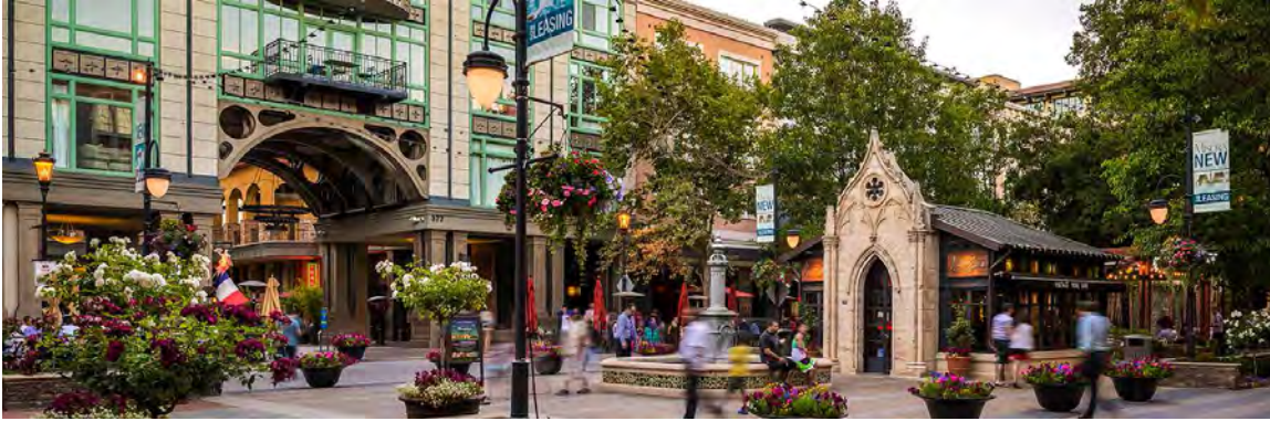
Santana Row: San Jose, California. A neo-gothic kiosk against a seeming iron truss. The development innovatively fuses retail, offices, and housing but seeks its expressive language in history. Tax credits, new zoning, new financial means: semiotic architecture.
