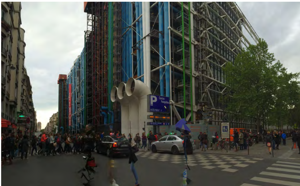
1971-73: the Centre Pompidou: an industrial aesthetic and a machine for art and culture. Sans actual production the factory is pristine four decades later. Photograph: Michael Bell.
