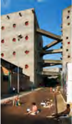
Figure 3. SESC Pompéia, São Paulo. View of the pedestrian bridge connecting old and new buildings.
