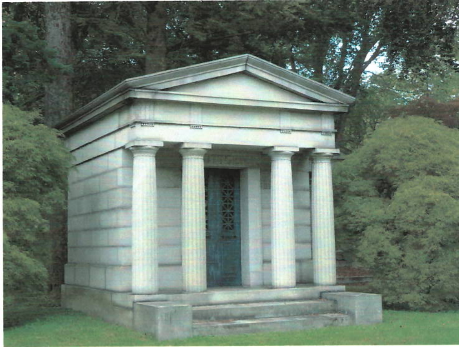
Fig. 10a: Lüttgen mausoleum, Chestnut Hill, Woodlawn Cemetery, Bronx, NY. C. E. Tayntor Granite Co. ca.1908. (Photograph by Max Yeston)
