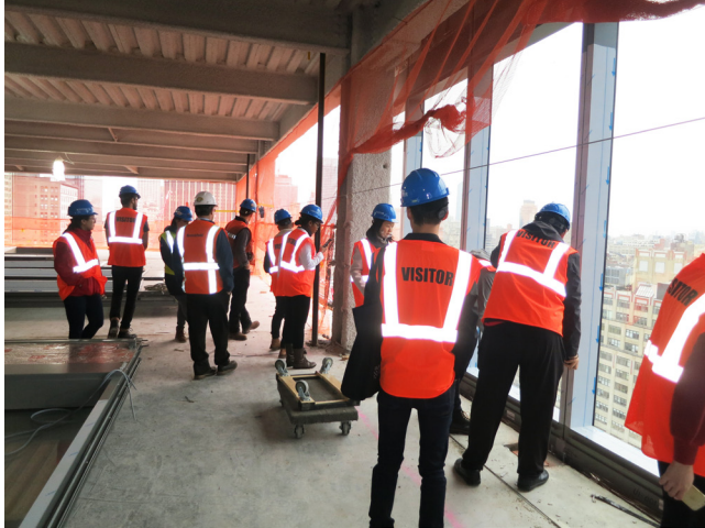
SITE VISIT TO MANHATTAN WEST NORTH EAST TOWER
