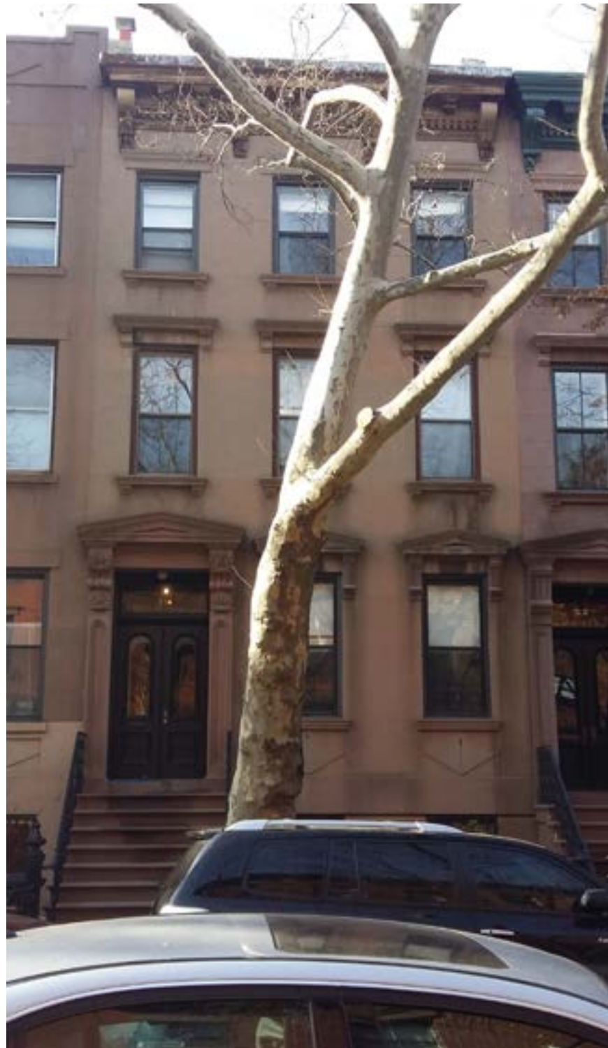
Fig. 2. Condition 2: Block 325 lot 36 source: Student Photo
