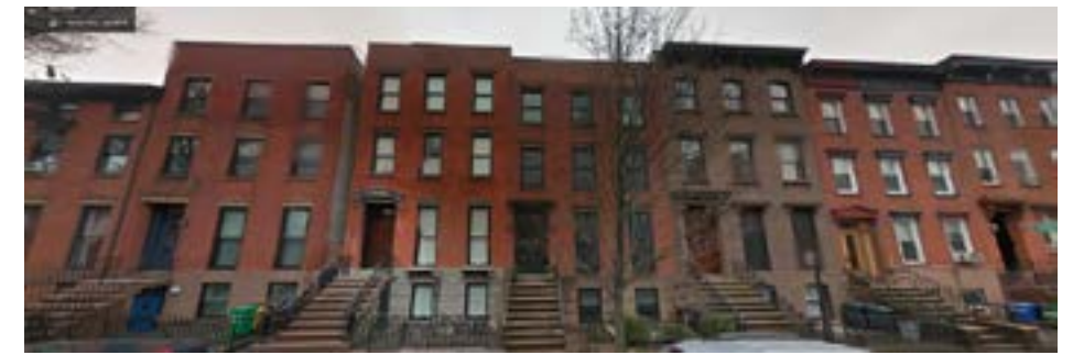
Block 332 source: Google Street view
