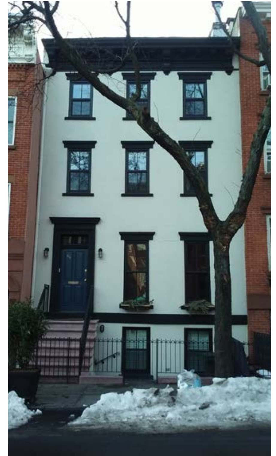
Fig. 3. Condition 3: Block 194 lot 17 source: Student Photo
