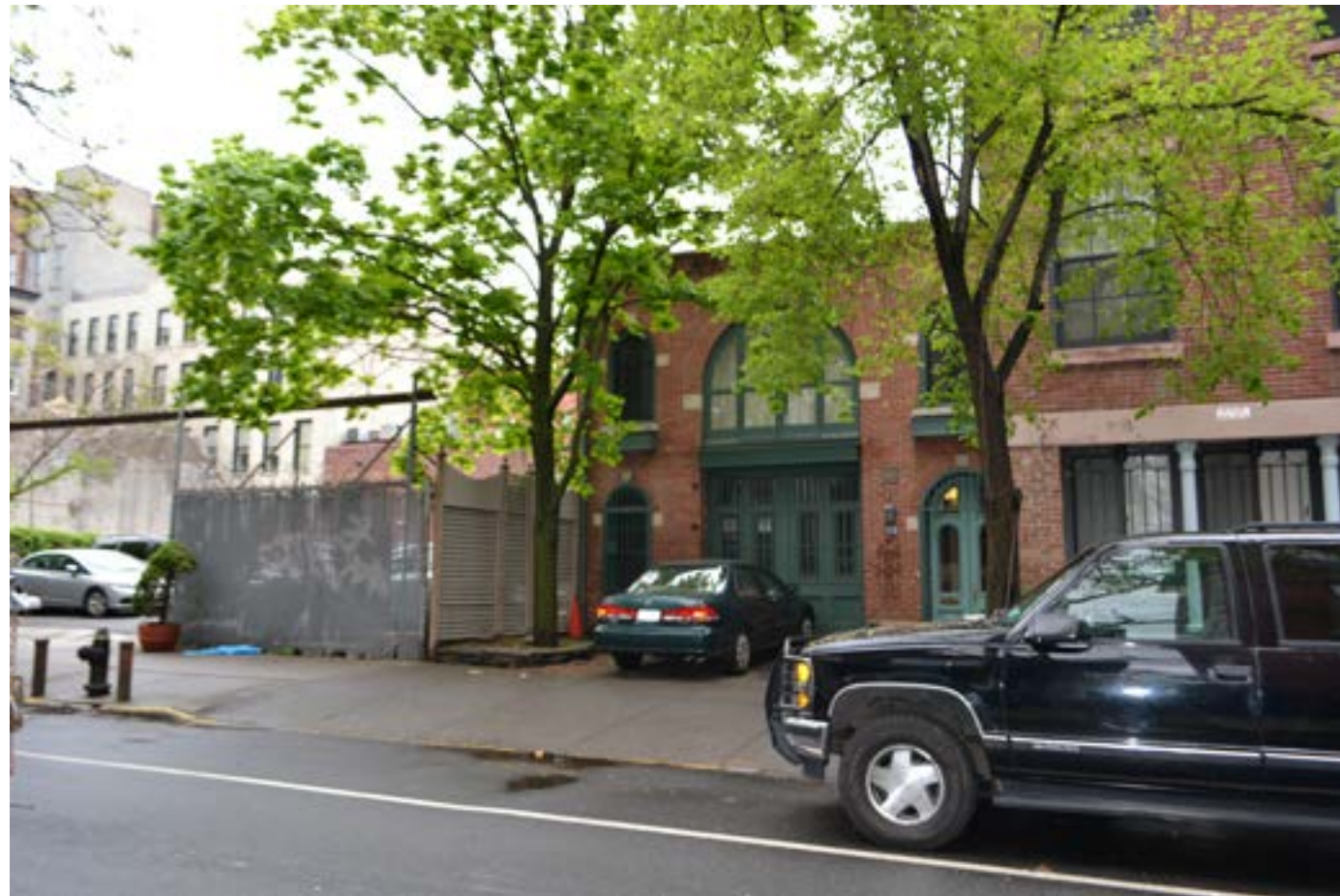
173 Pacific Street source: student photograph
