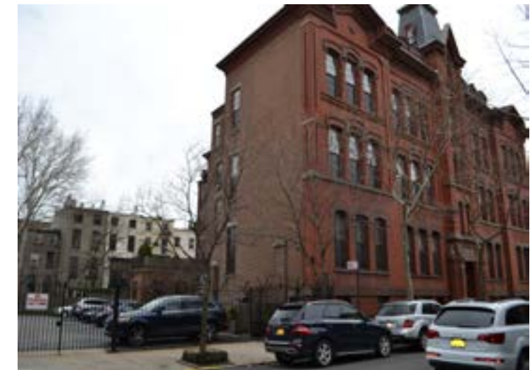
Site 2: 188 Pacific Street Source: student photo
