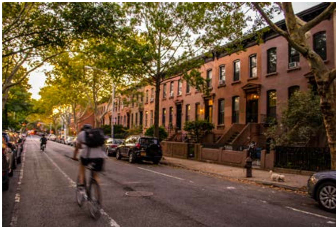
Wyckoff Street Italianate Row Houses Source: student photograph
