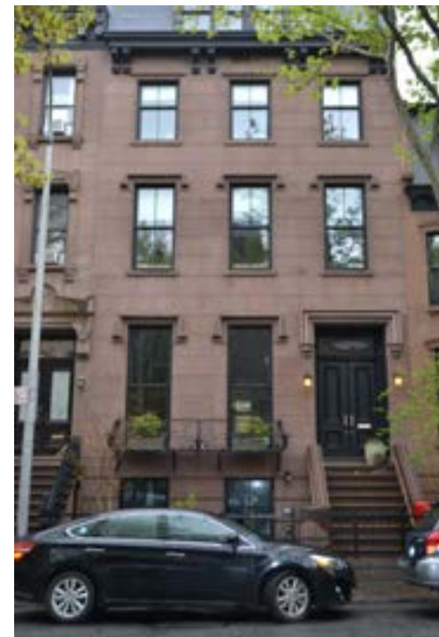
374 Pacific Street source: student photograph
