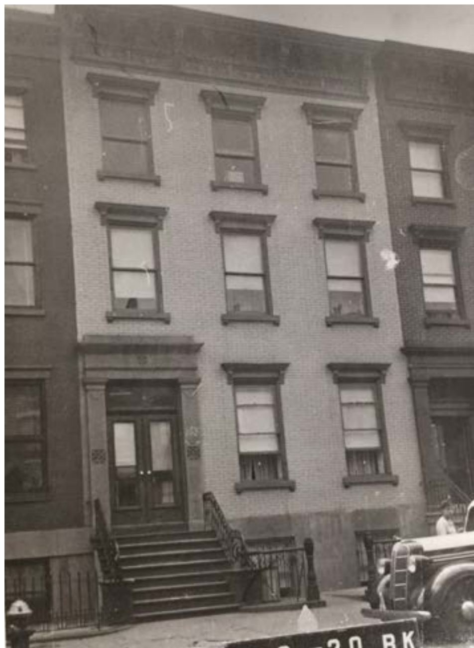
1930's / 1940's Photograph Source: nyc 1930-1940s tax photographs
