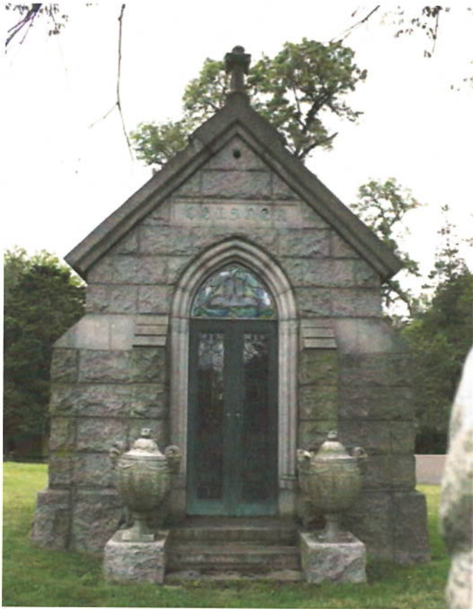
Figure 2: Oelsner Mausoleum Front Facade
