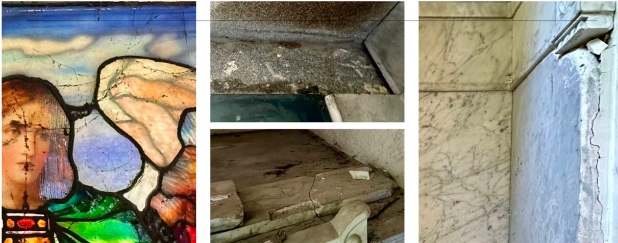
(Figure 6. General conditions)
