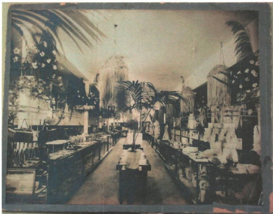
First Floor of the Bon Ton store, 1910, (Lebanon County Historical Society).
