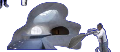
SHOTCRETE a construction technique invented by Carl Akeley for sculpting taxidermy, used in the new Glider Center
