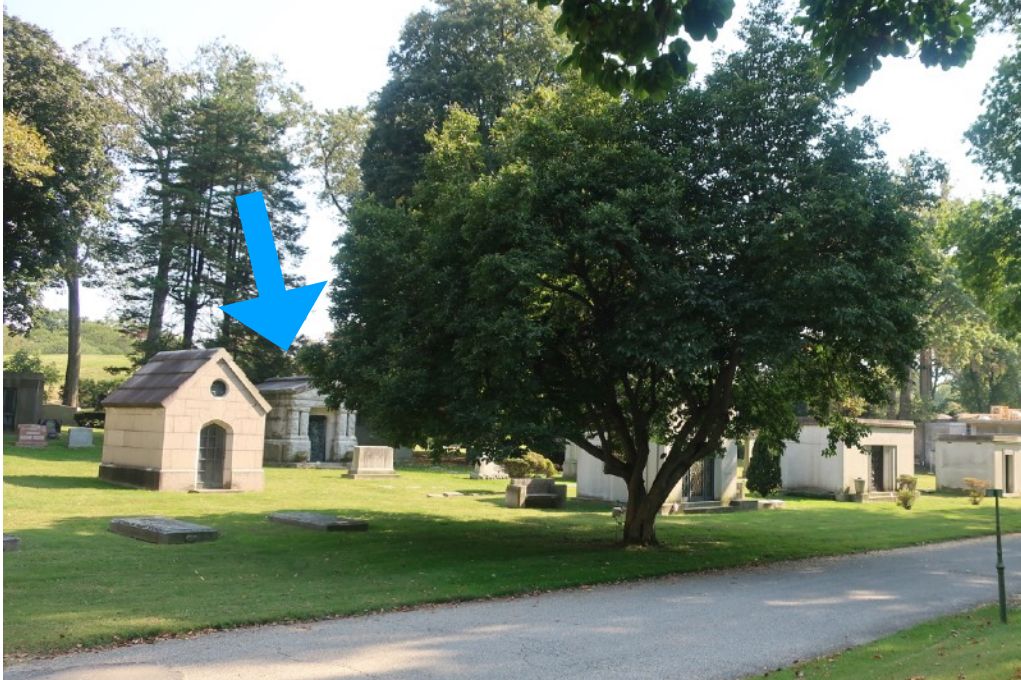
Fig. 3: Truss mausoleum as approached from Myosotis Avenue.
