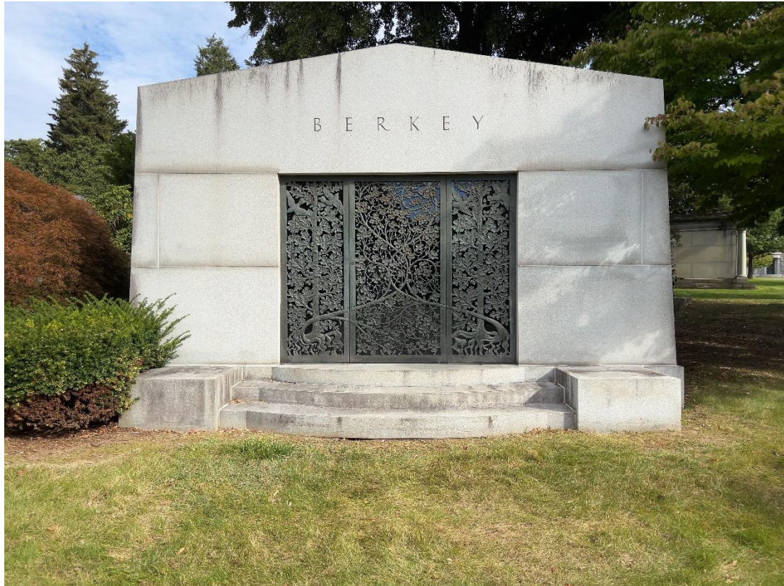
Figure 1: South Elevation. Source: Author
