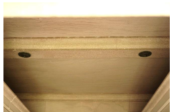
25 Beam on the ceiling
