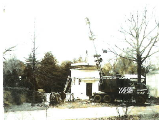
Construction: Photos obtained at H.K. Peacock Memorials Office
