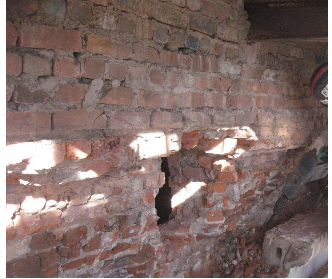
BRICK MASONRY WALL
