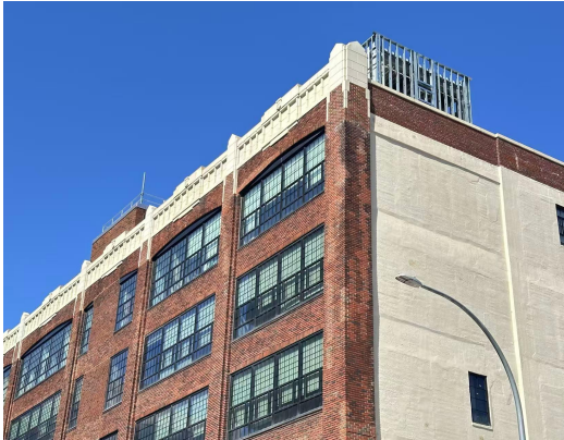
Site visit and measurements Photo from Zhi Yang, March 24, 2026
