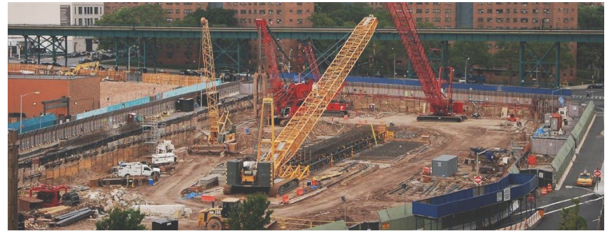
DEMOLITION AND REPLACEMENT
