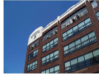
Restoration works of some spaces under Columbia University
