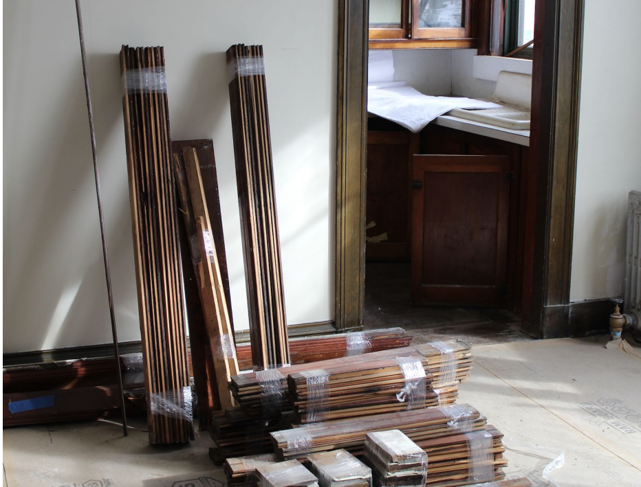
DECONSTRUCTION AND SALVAGE OF BUILDING MATERIALS
