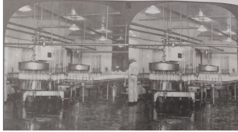
Borden Milk Processing Plant
