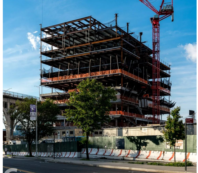
EMBODIED CARBON - CONSTRUCTION OF COLUMBIA BUSINESS SCHOOL
