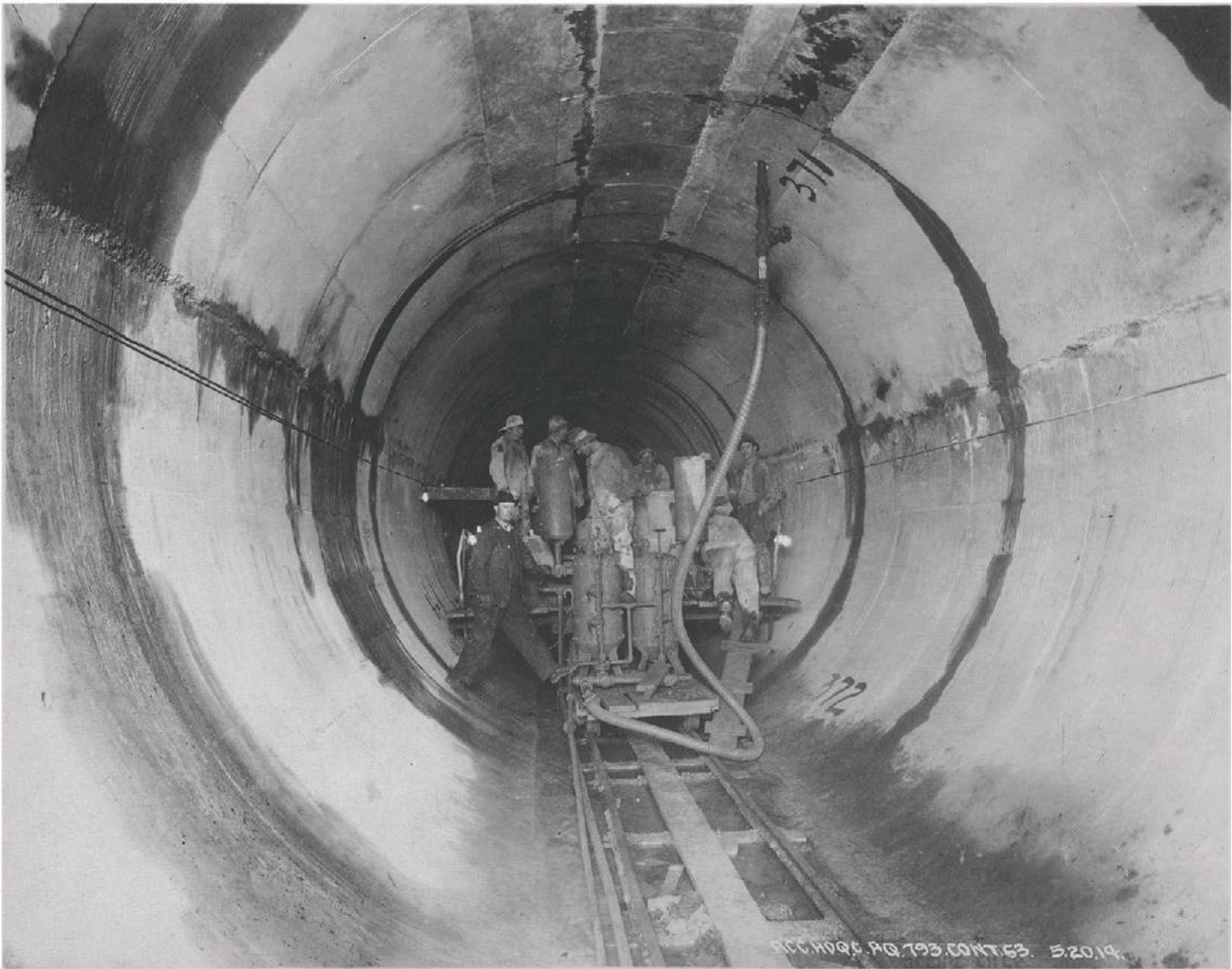
NYC Water Tunnel n. 1, circa 1914.
