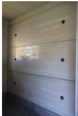
Interior South Elevation of Essig-Foeller Mausoleum
