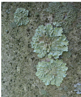
Detail: Biological Growth on Essig-Foeller Mausoleum Urn
