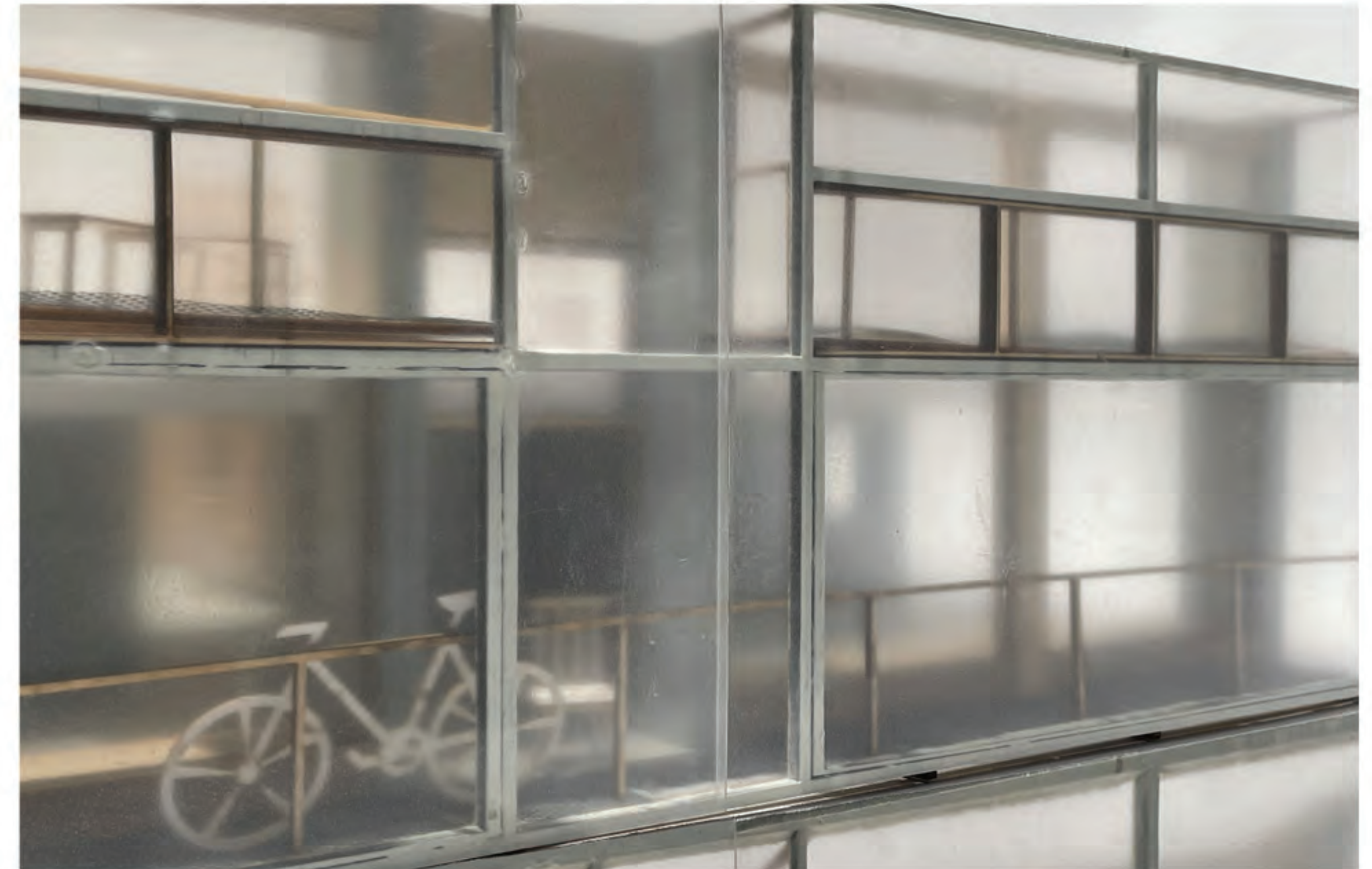
City-facing Double Facade System with Sliding Partitions
