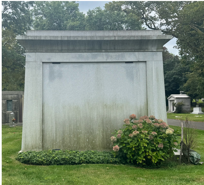
Figure 6: Lindsey Johnston, North Elevation, 2025
