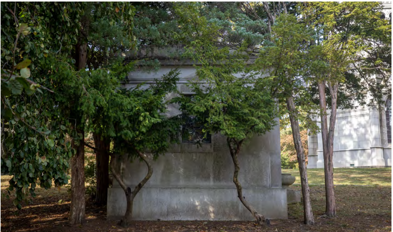
Fig. 31 Creighton Family Mausoleum, Rear Facade, Woodlawn Cemetery, Bronx, New York, NY. Photograph by Khaled Alanjery, October 2025.
