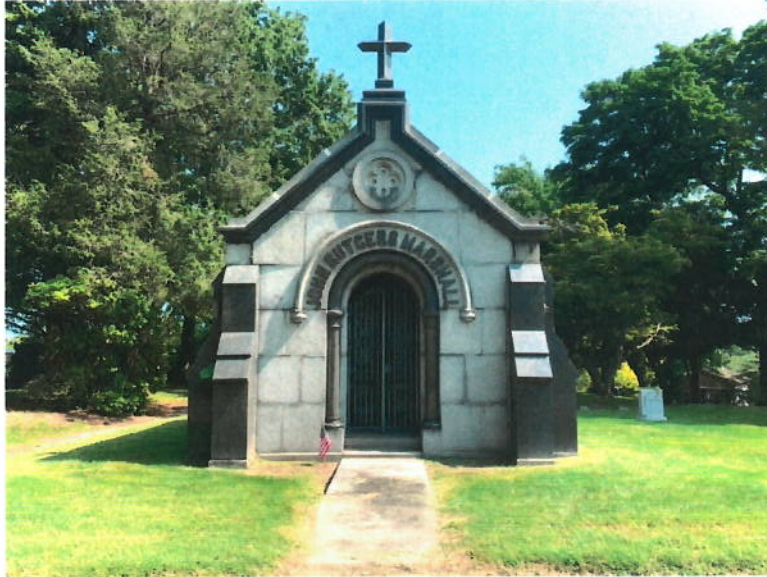
Figure 2 The Primary Façade of the Marshall Mausoleum 25
