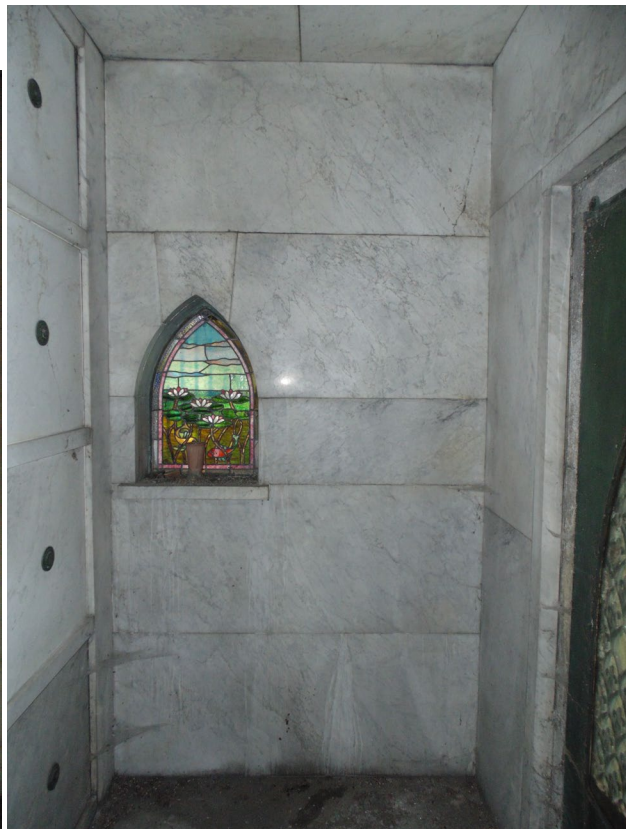
Figure 10: West window interior
