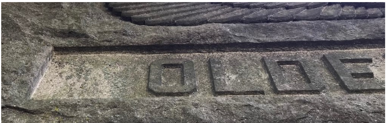
Figure 18: Recessed lettering with stone cut layers visible
