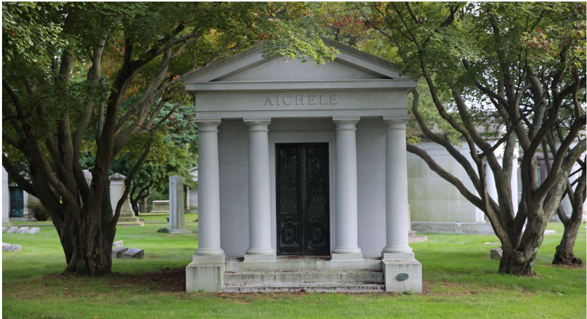
Front view of the Aichele Mausoleum showing steps, buttresses, doric columns, pediments, walls, and roof in barre granite.
