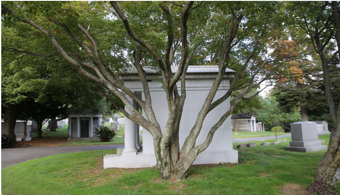
West elevation of the Aichele Mausoleum, showing the roof stone in one piece with a small cap on top.
