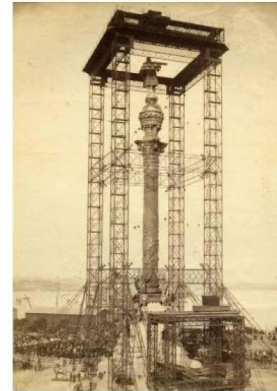
Figure 3. Construction of the Columbus Monument in Barcelona, 1888.
