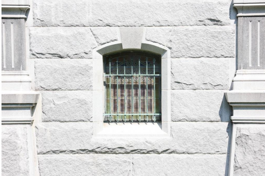
Figure 18: The exterior view of the window
