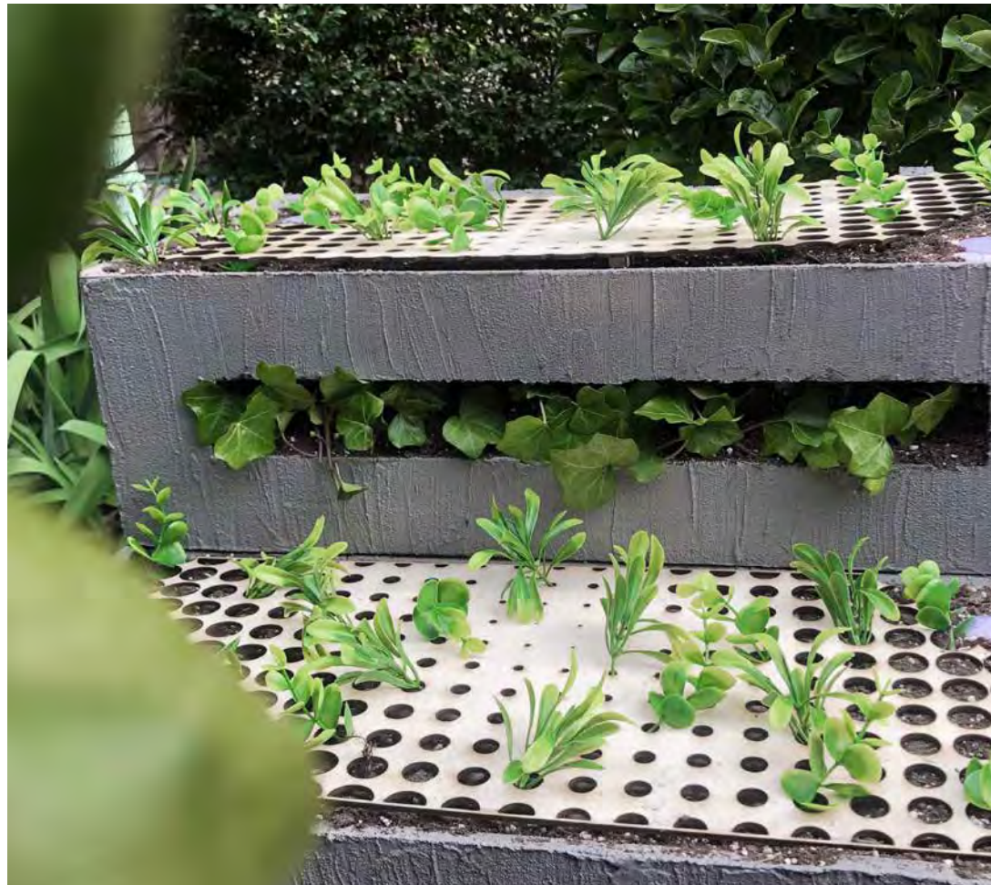
1:1 Scale Detail Model of Step Planters
