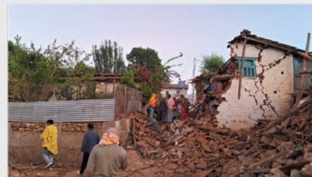
Hundreds of homes destroyed in the most recent large scale earthquake in west Nepal. November 2023.
