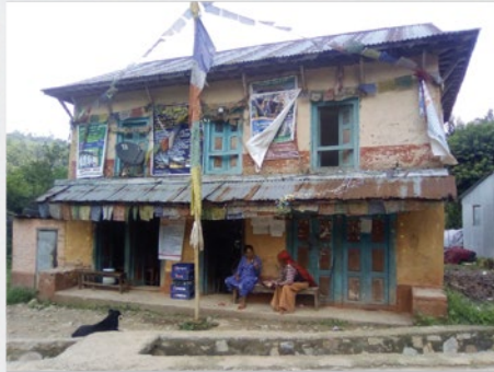
Typical Nepali single family house: Constructed primarily with stone walls, these houses feature roofs fashioned from materials such as thatched grass, zinc, or tin. Occasionally, the walls are adorned with a coating of clay and manure. Additionally, wooden pillars reminiscent of log cabins support these structures. Many of these traditional houses suffered damaged in the large earthquakes.
